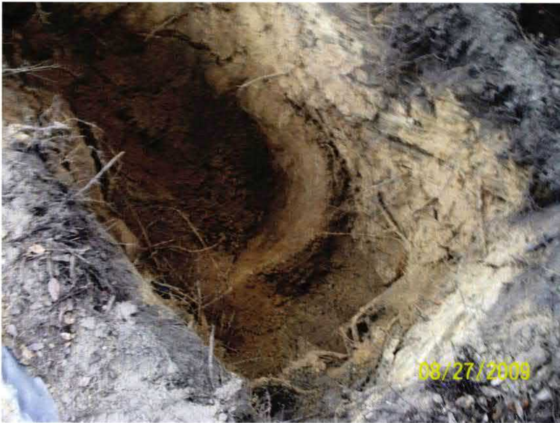
Picture 1: UST 1237Dove excavation after tank removal.
