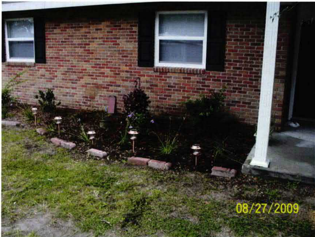
Picture 2: UST 1237Dove site after completion of work.
